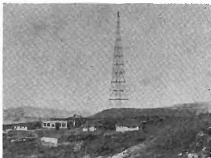
Situated in a very remote and lofty position at Gebbies Pass, 18 miles from Christchurch, New Zealand. 3YA is a favorite mark for American DXers. The programs are relayed by wire from the studio in the city. One of the two 300-foot towers is shown in the photo.
